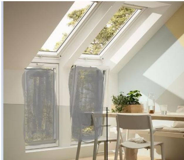
Example combination window unit with image showing extent of obscure glazing
